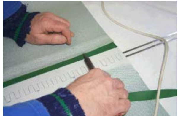
Add a small film to fill the gap and fix it with hot points
